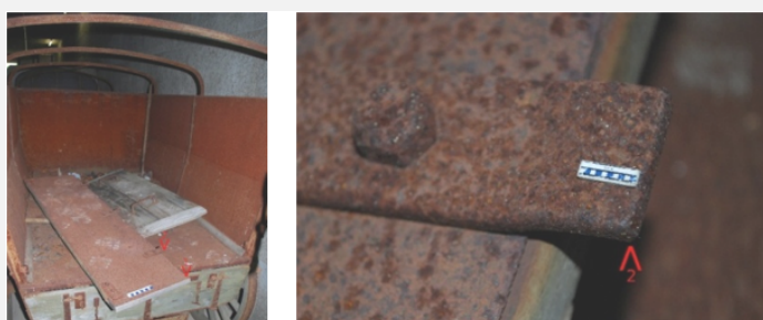
Fig. 1: Fitting on back panel of a military carriage,
