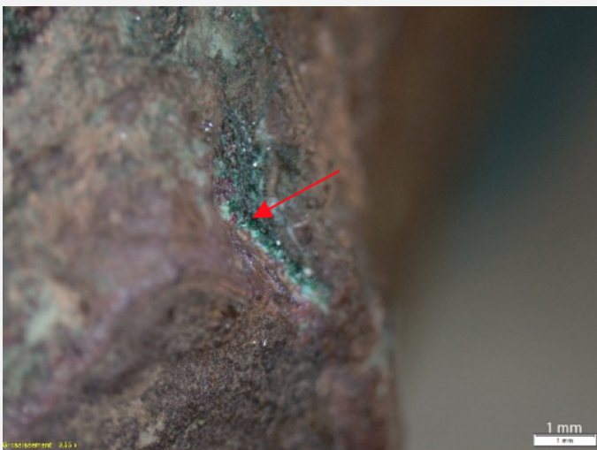
Fig. 13: Observation of the dark green corrosion product,
