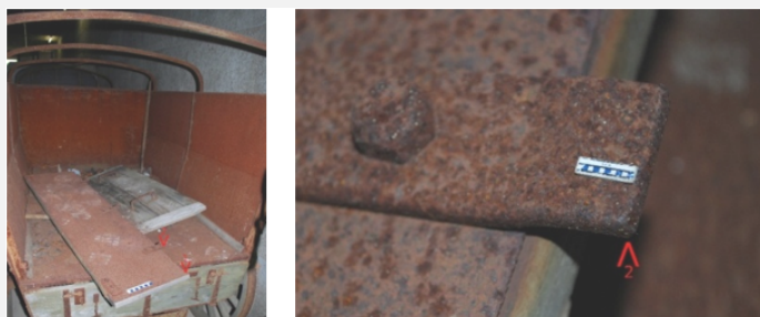
Fig. 1: Steel fitting on back panel of a military carriage (©Tarchini),
