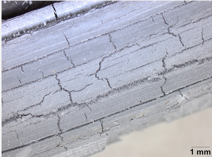
Fig. 4: Detail of the corroded lead came
