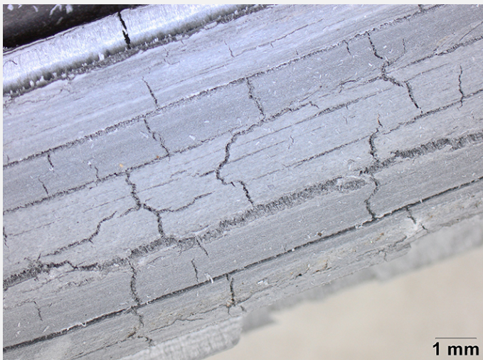
Fig. 4: Detail of the corroded lead came
