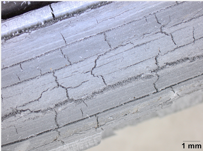
Fig. 4: Detail of the corroded lead came
