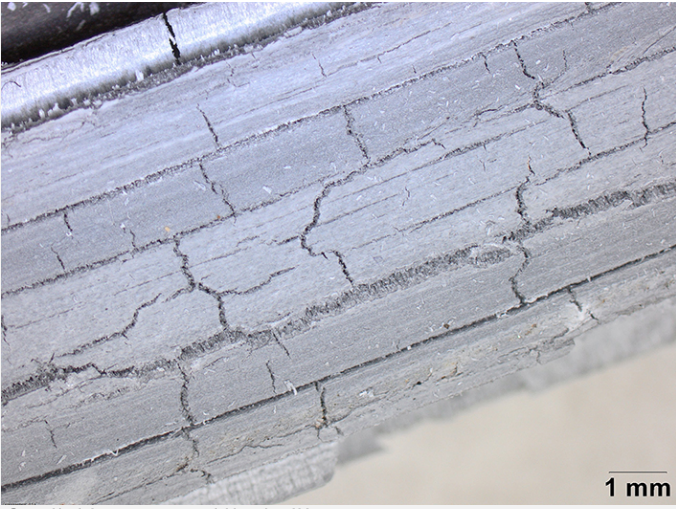
Fig. 3: Detail of the corroded lead came,
